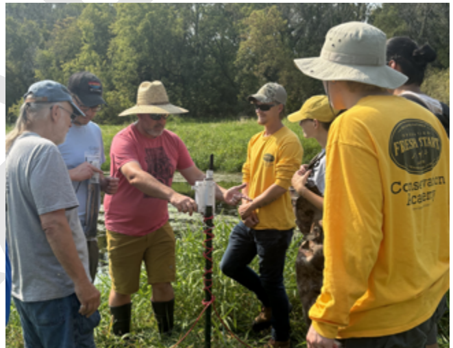
OPERATION FRESH START CHLORIDE MONITOR INSTALLATION
