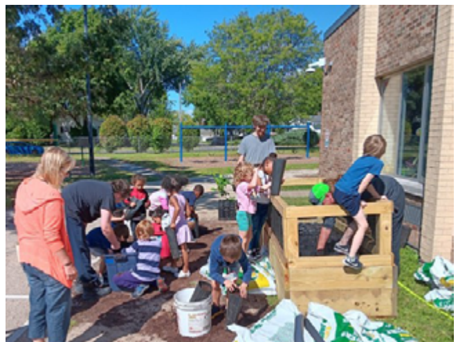
TREE CRIB INSTALLATION AT WESTSIDE ELEMENTARY IN SUN PRAIRIE
