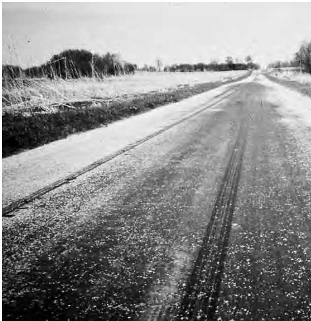
▼ Severe flushing.
