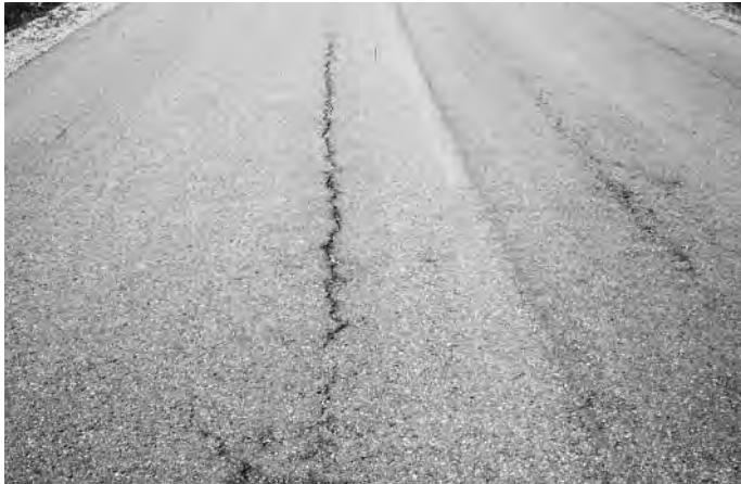
Multiple open, longitudinal cracks that are raveling. ▼
