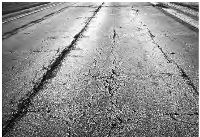
Multiple open, longitudinal cracks that are raveling. ▼
